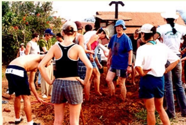
Learn by doing: superadobe construction at Ecoversidade
